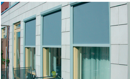
Exterior Solar Screens
